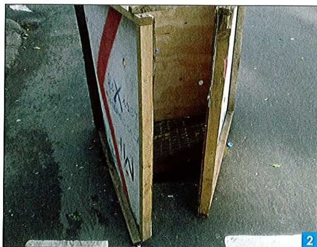
An isolated and signaled manhole with a considered high flammable gas concentration, waiting for repairs.
