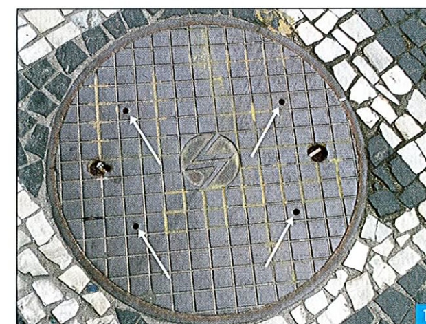
These holes cut into manhole covers are intended to aid in the release of gas buildup.
