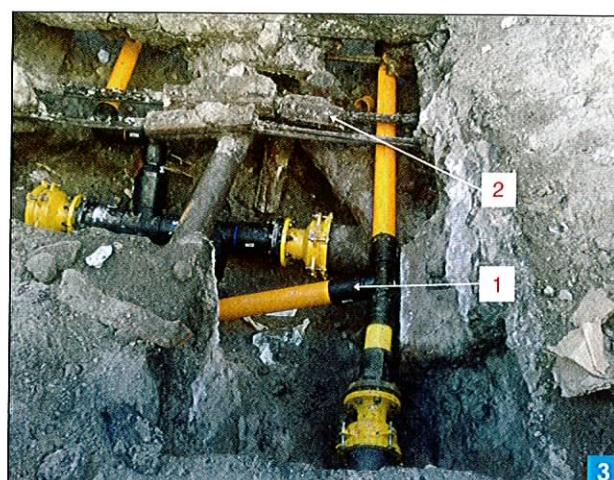
An excavation of the damaged terracotta ducts of the street lighting circuits: 1) new polyethylene gas piping and 2) damaged terracotta ducts exposing the street lighting cables.
